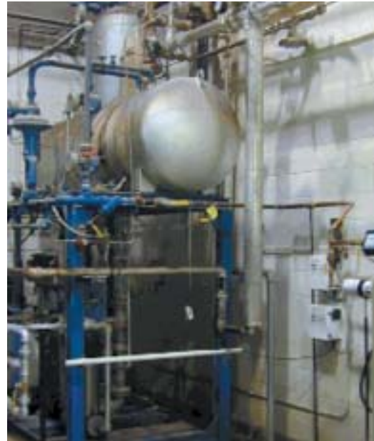
Deaerator Tank for 500HP Boiler Using Dolphins
